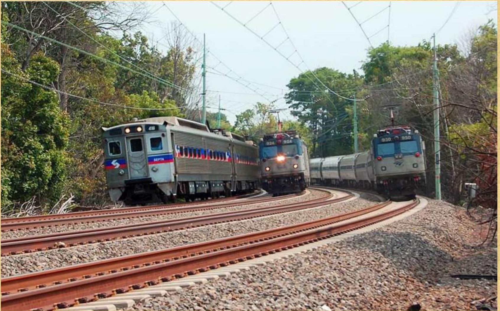
Curve with superelevation
