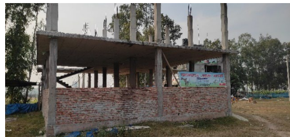
Affected Building under Construction
